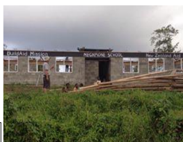
Megamone Classrooms in the process of being built!
